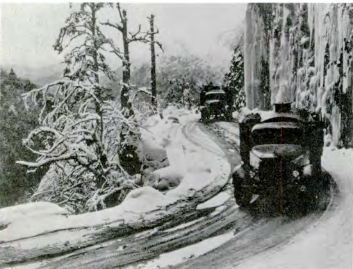
Army trucks on the Szechwan-Tibet road. This is a soil-aggregate type of construction, classified as a loose-surface, all-weather road. Constant maintenance, including snow removal, is required to keep this main access road to Tibet open to traffic.
