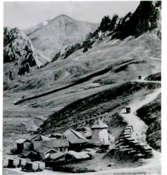
Station on the Szechwan-Tibet road. This road, like most of the main roads in western China, stretches for hundreds of miles through sparsely inhabited areas. Rest, refueling, and supply stations, constructed about one day's drive apart, vary in size and services offered, and often accommodate road maintenance crews. The station shown here is one of the larger and more complex ones.
