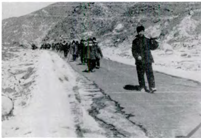
Road from Peking to the Great Wall, Hopeh Province. Only a few thousand miles of roads in China have high-grade surfaces such as the bituminous-treated surface here. Road surfaces may vary from section to section; this road, for example, has a concrete surface in the vicinity of Peking, although concrete surfaces are rare in China. Near oil refineries, residual oils or tars are applied to harden or stabilize the surface.
