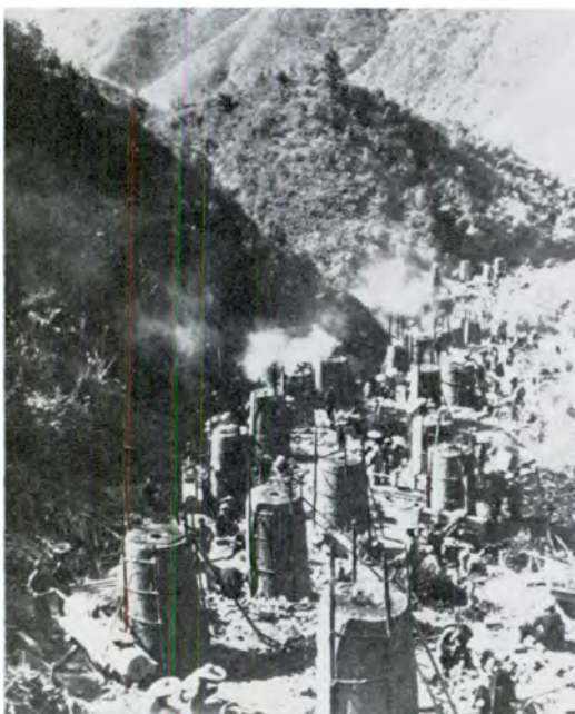
Native copper smelting furnaces in Southwest China. Furnaces such as these flourished during the 18th and 19th centuries furnishing copper for the imperial mints in Peking. During the Leap Forward (1958-60), similar primitive "backyard furnaces" were built by the thousands—principally to produce pig iron.
