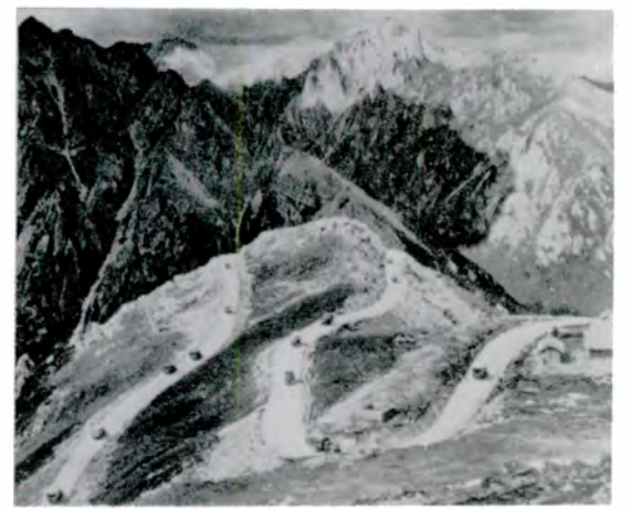
Road in western China. Looping precipitous roads, such as this one, are common throughout the mountainous country of China. Road loops are often so numerous that road mileage is doubled or tripled compared to the "crow-fly" distance. Mountains in eastern China, although not as high as those shown here, often are as rugged and as troublesome for construction, maintenance, and transit.
