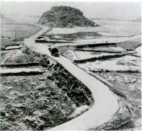
Roads in Kweichow Province. Roads in low-lying areas are built on levees. This road is typical of those found in the principal plains and basins of eastern China.
