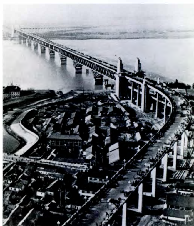
Yangtze river bridge at Nan-ching. This bridge, opened to rail traffic in 1968, carries a roadway on its upper deck and a double-track railway on its lower deck. A strategic link on the important Peking to Shanghai rail line, construction continued during the turmoil of the Cultural Revolution. This bridge is the third across the Yangtze; the others are near Ch'ung-ch'ing and Wu-han.
